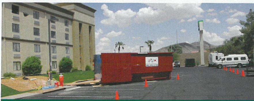
On the left part of the image, you can see plywood protecting the landscaping and lawn when crews tossed down debris for the large dumpster.
