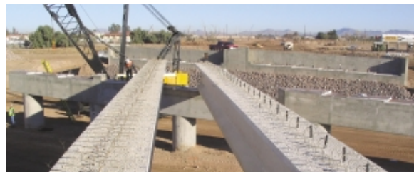
Ellsworth Loop Project, Queen Creek
